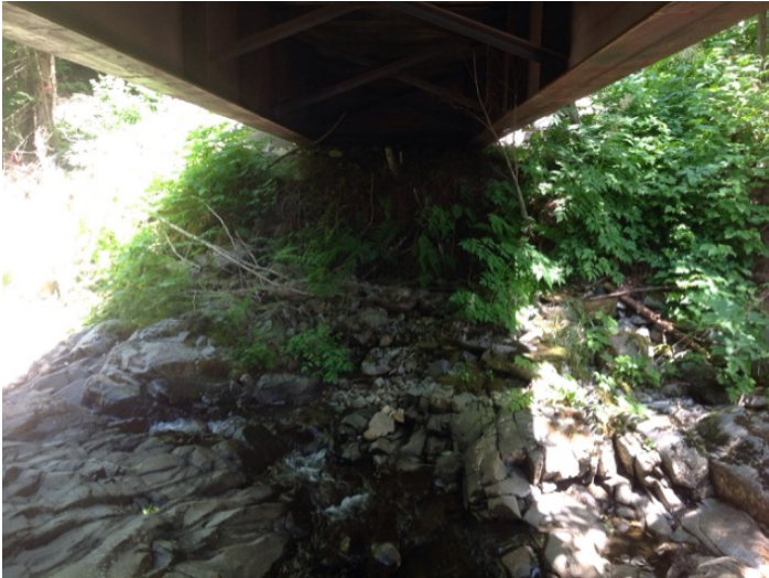
Left Bank Abutment when facing downstream
