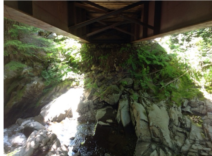
Right Bank Abutment when facing downstream
